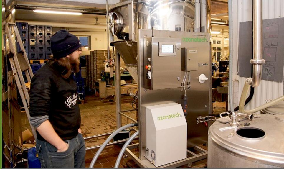
The RENA Vivo A-series system is connected to tanks and other process equipment during CIP sanitation. The brewmaster Johan Hansson is observing the system during operation.
